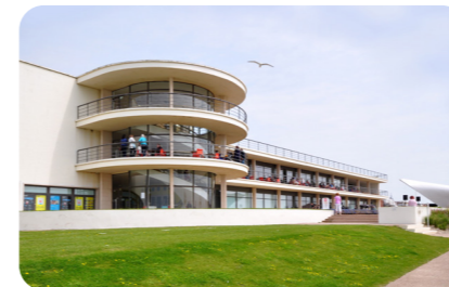
De La Warr Pavilion, England
